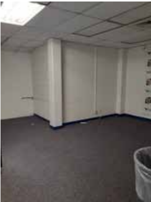
Dressing Room 3 Entrance View
